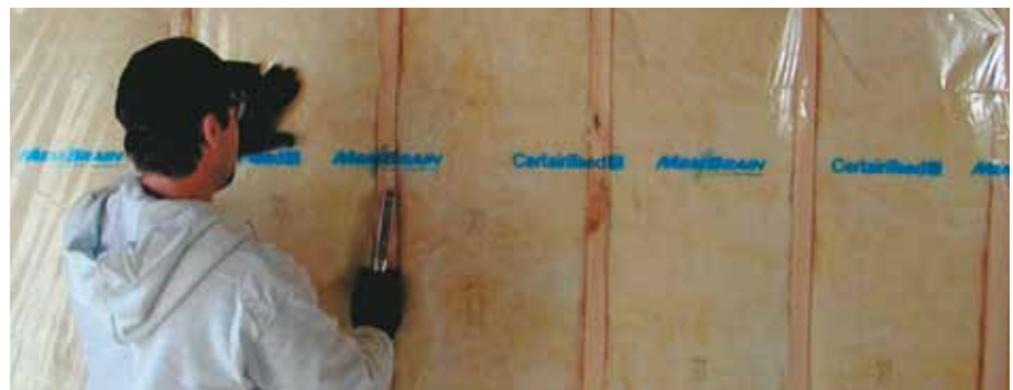
Molecular-scale pores close under dry conditions, blocking vapour transmission.
